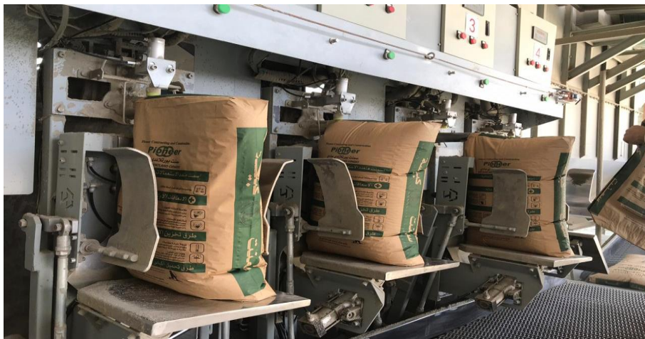
Figure 1.4. Three pictures from the Al-Kubaisa cement factory.
